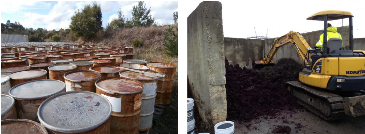
Figure 3: Photographic examples of closed systems: drum storage of contaminated industrial solid waste awaiting batch treatment in Tasmania, Australia (left); treating a batch of contaminated industrial soil within a bunded handling area in Melbourne, Australia, (right).
